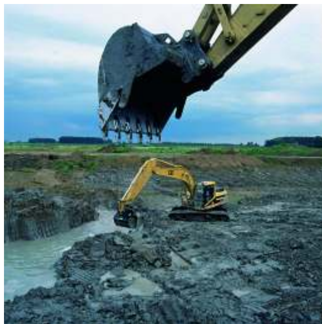
Figure 16. Lowering the floodplain provides more storage for flood water.
